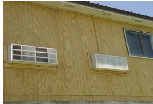
Lender Required Repairs / RUSH
