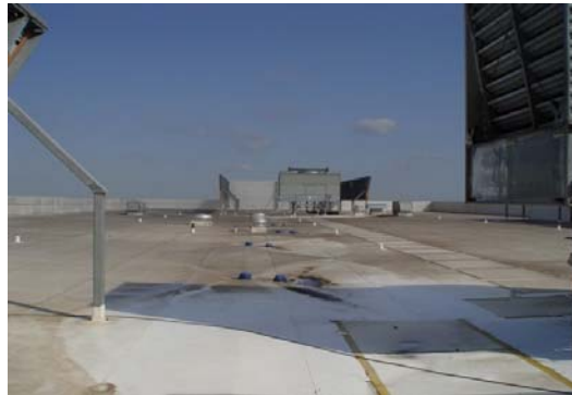
Mechanical Room & Roof
